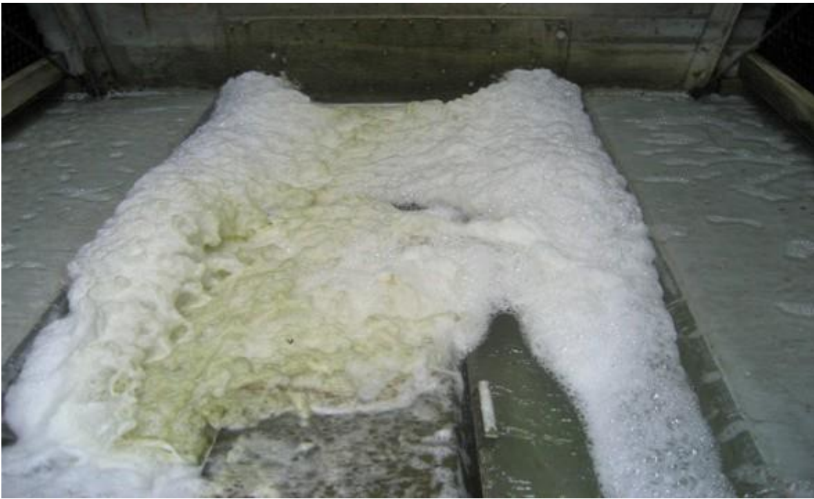
Water, foam, and organic contamination before starting on ProMoss™
