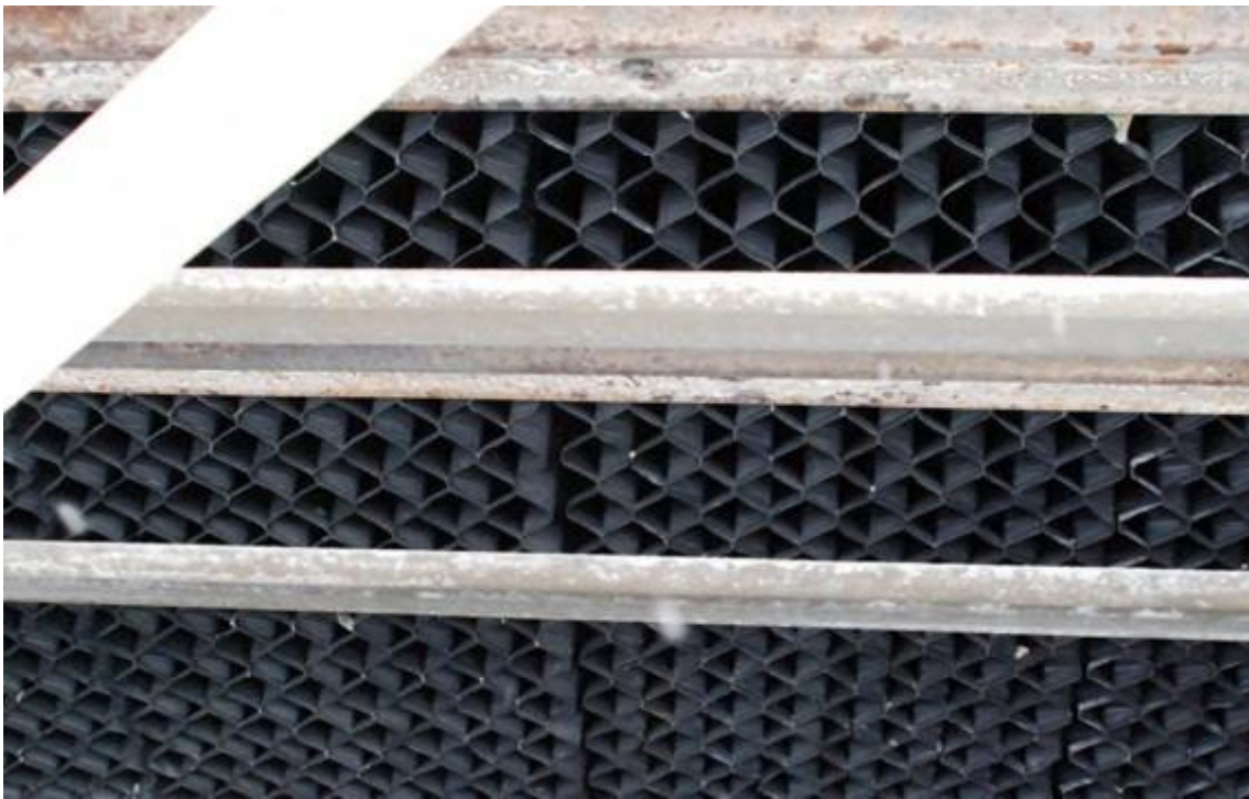
Cooling tower media from 16 year old phase one test facility after two cooling seasons on ProMoss™
